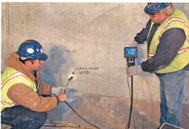
Inspection of a void in a grouted post-tensioning duct using a borescope. Photo: Structural Technologies.
