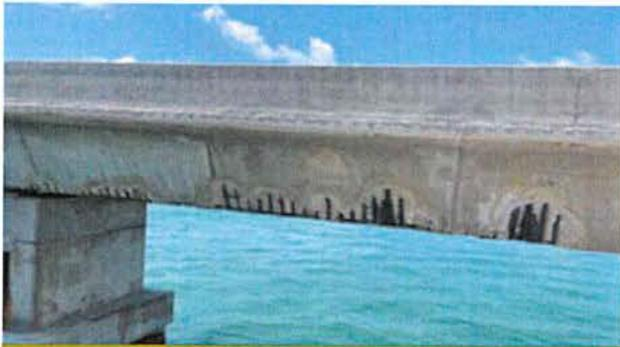
A precast concrete segmental bridge with loss of concrete cover and reinforcement cross-sectional area due to corrosion of reinforcement after approximately 45 years of service and exposure to a saltwater environment. Photo: Finley Engineering Group.
